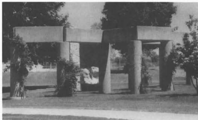
Tom Sternal, Pavillion , 1993. Reinforced concrete, marble, sandstone, wisteria and virginia creeper vines, 12.5 x 30' (3.8 x 9.1 m). Photo: Katherine Stewart.
